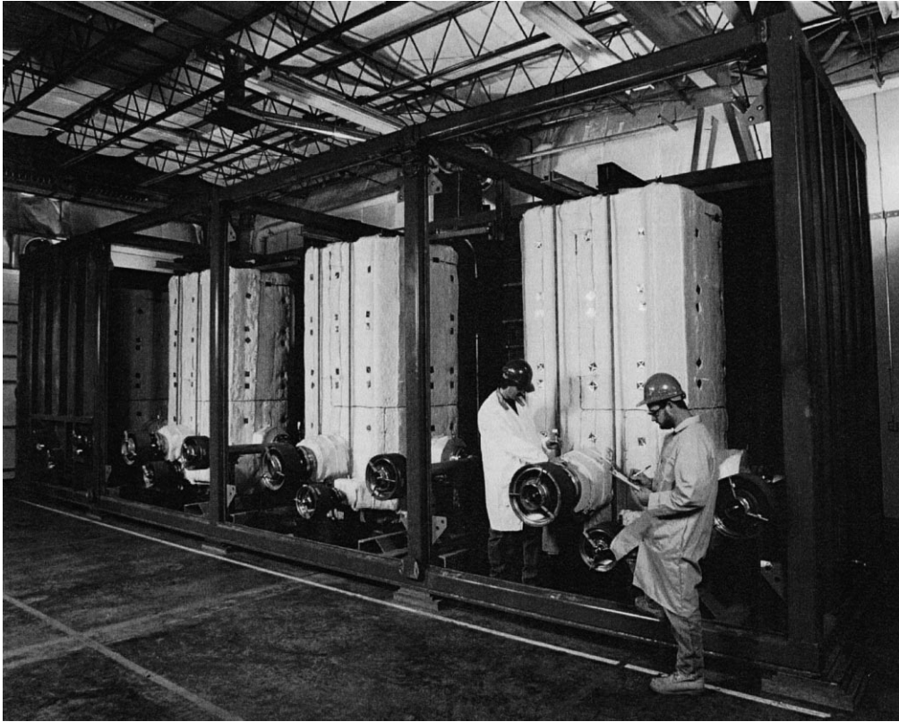
Fig. 4. Four-stack 500-kW DFC™ module under construction at FCE.
